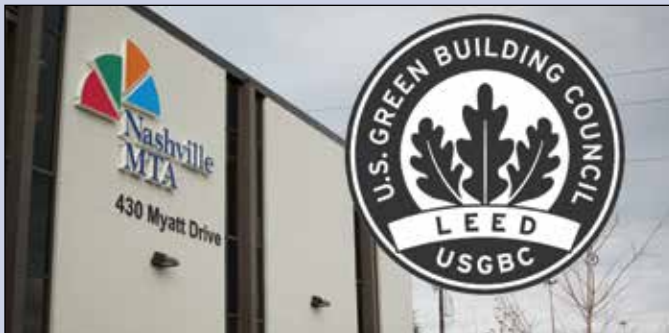
MTA Myatt Drive facility
